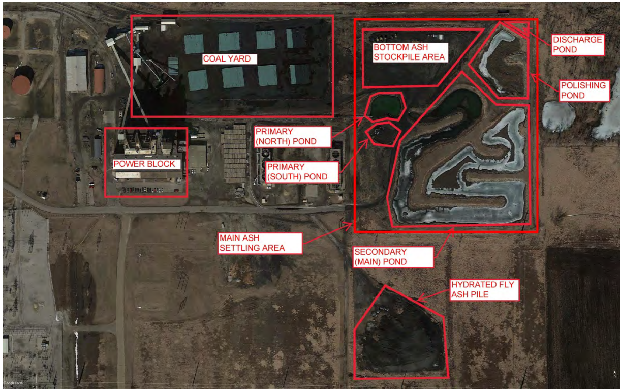
Figure 1 – Current Layout of Sutherland Generating Station (Prior to Closure)
