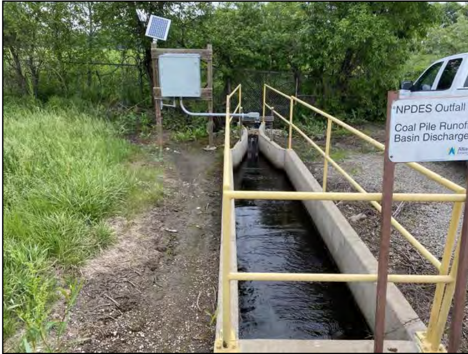
Photograph C-35: View of existing outfall feeding intermittent S-3 at PP-5, facing north.
