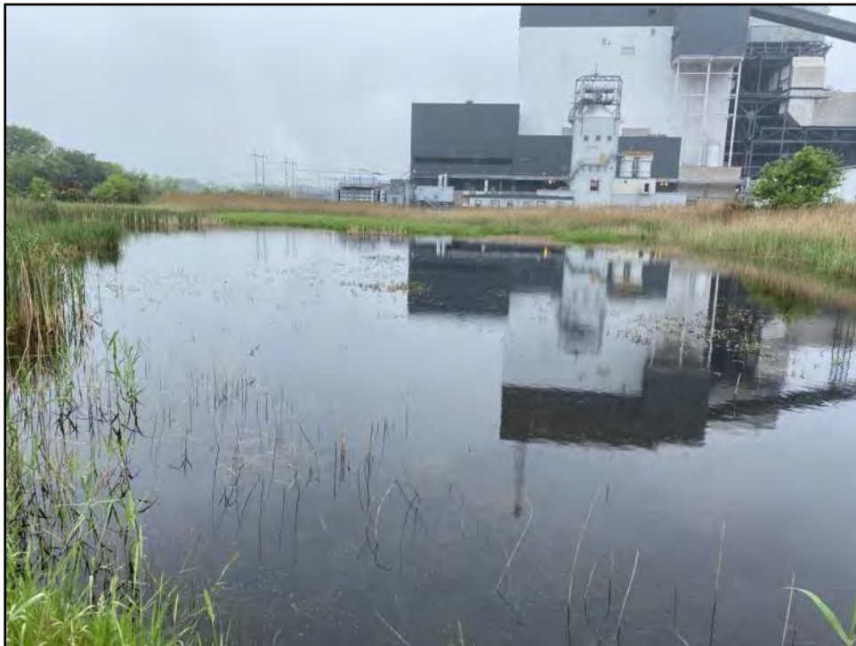
Photograph C-24: View of PUB W-11, facing west.
