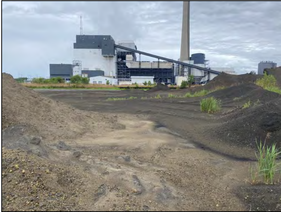
Photograph C-37: View of representative spoils area within bottom ash area at PP-11, facing west.
