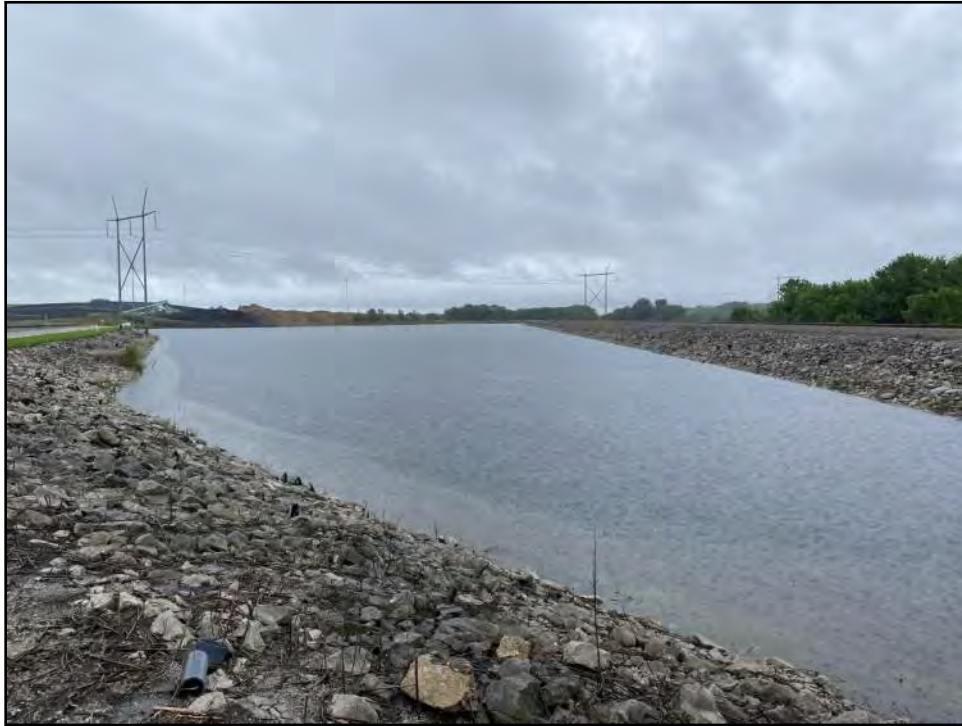
Photograph C-27: View of PUB W-15, facing northwest.
