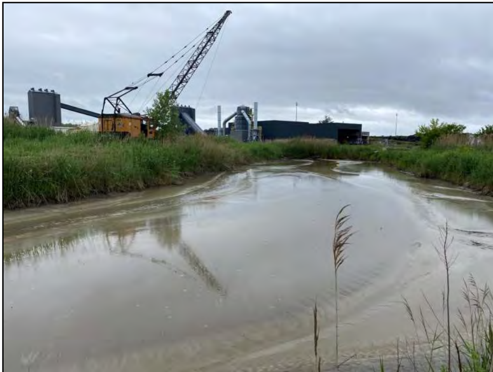
Photograph C-26: View of PUB W-14, facing northwest.
