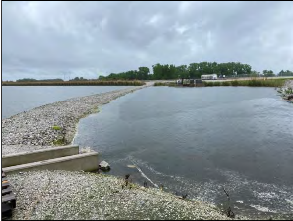
Photograph C-25: View of PUB W-13, facing north.
