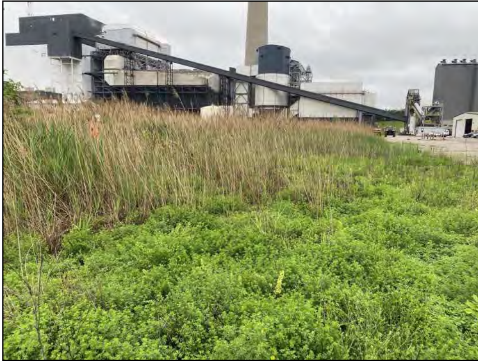
Photograph C-19: View of upland SP-19, facing west. A soil sample was not collected.
