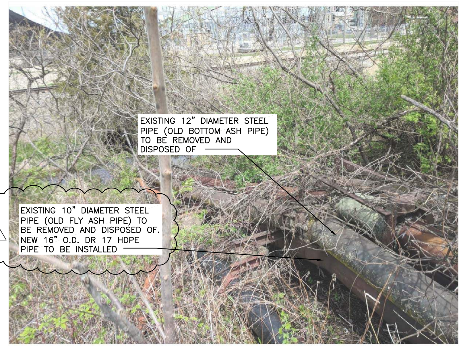
PHOTO DETAIL NORTH SIDE OF CMP CULVERT NTS
