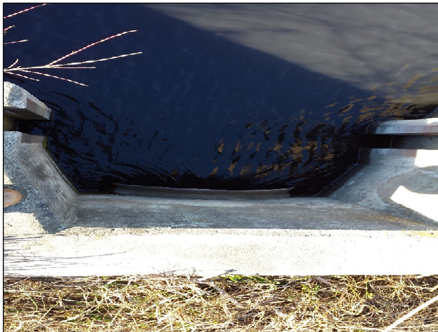
Photo 8: Outlet of EDG B-Pond hydraulic structure. Water from EDG B-Pond discharges into the EDG C-Pond. Water within EDG C-Pond flows to the east to the EDG F-Pond. Water in the EDG F-Pond discharges through the facility's WPDES Outfall 004 into Lake Michigan.
