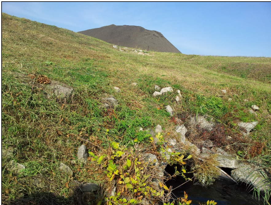
Photo 6: Outlet of 48-inch diameter corrugated metal pipe which contains flows of the EDG Slag Pond and EDG South A-Pond. The water discharges into the EDG B-Pond.
