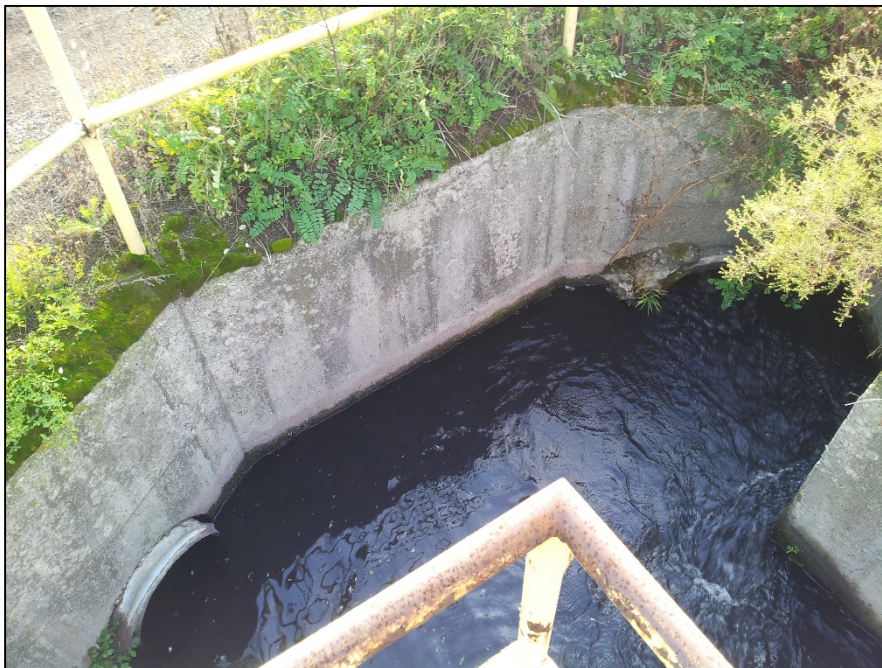
Photo 4: Outlets of EDG North A-Pond and EDG South A-Pond hydraulic structures. Currently, water only flows through the hydraulic structure of the EDG South A-Pond. Water flows through a Parshall flume structure and into a 48-inch diameter corrugated metal pipe.
