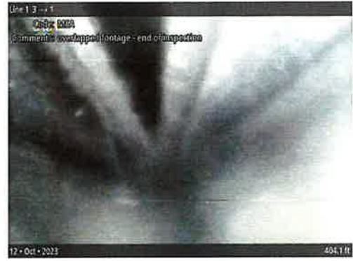
MSA at 404.1 ft | overlapped footage - end of inspection
