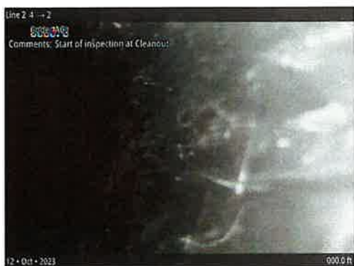
ACL at 000.0 ft | Start of inspection at Cleanout
