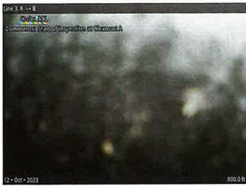
ACL at 000.0 ft | Start of inspection at Cleanout A
