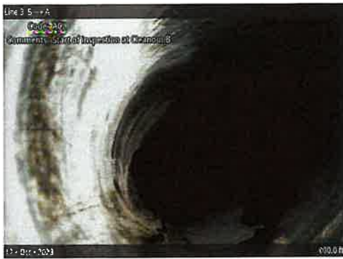
ACL at 000.0 ft | Start of inspection at Cleanout B
