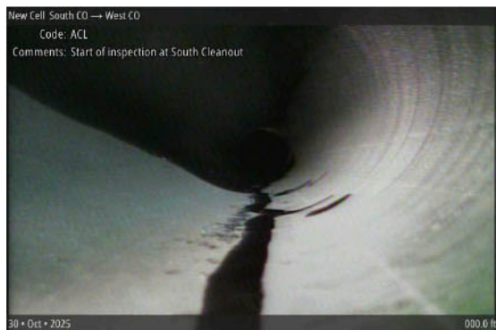
Access Point - Cleanout Landfill at 000.0 ft | Start of inspection at South Cleanout
