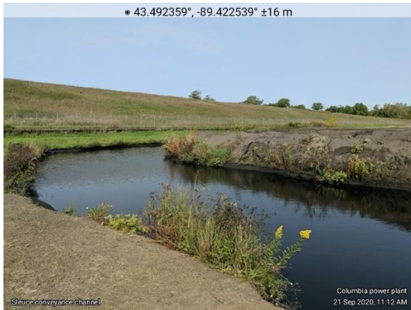
Photo #7 Water Conveyance Swale
