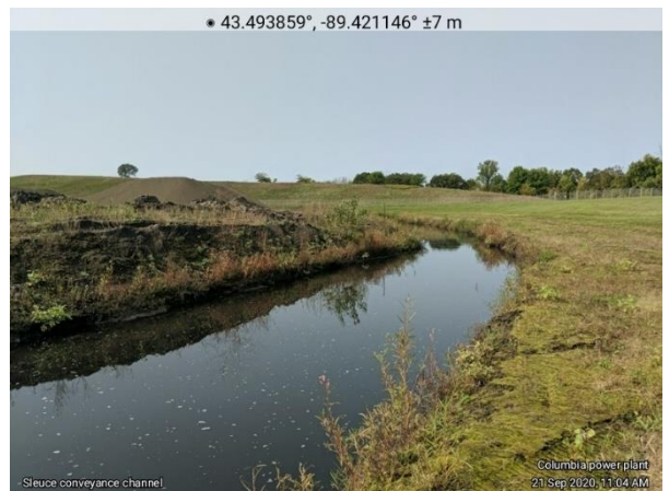
Photo #6 Water Conveyance Swale
