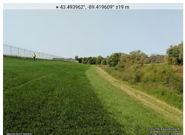
Photo #12 Northern Berm and Wetlands to North.
