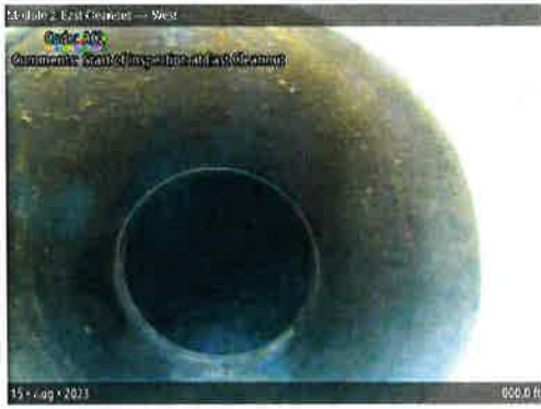
ACL at 000.0 ft | Start of inspection at East Cleanout
