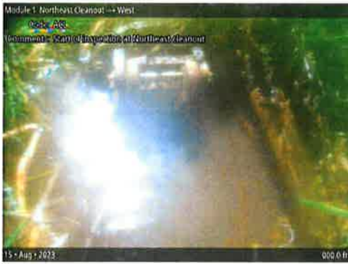
ACL at 000.0 ft | Start of inspection at Northeast cleanout
