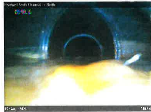
MGO at 140.5 ft | Crossover
