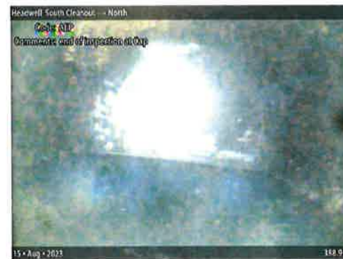
AEP at 388.9 ft | end of inspection at Cap
