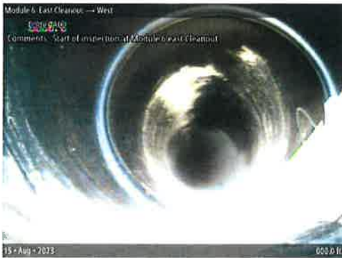
ACL at 000.0 ft | Start of inspection at Module 6 east Cleanout
