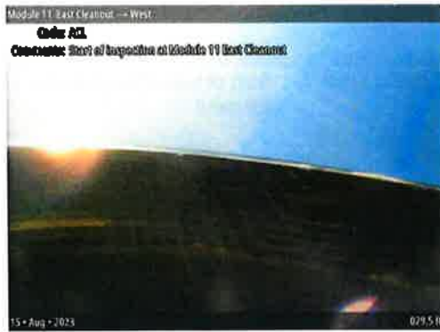
ACL at 000.0 ft | Start of inspection at Module 11 East Cleanout
