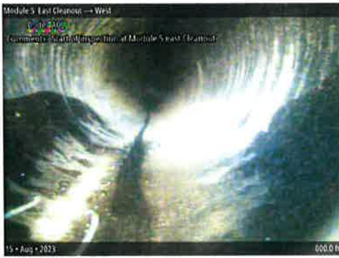
ACL at 000.0 ft | Start of inspection at Module 5 east Cleanout
