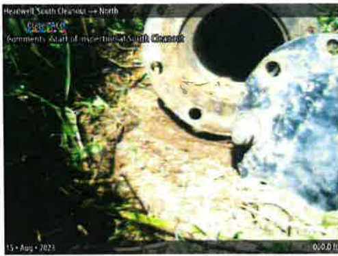
ACL at 000.0 ft | Start of inspection at South Cleanout
