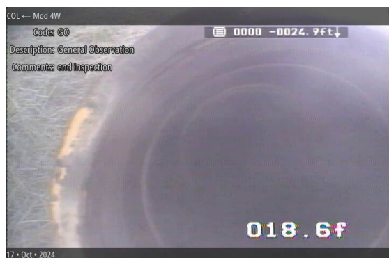
General Observation at 000.0 ft | end inspection
