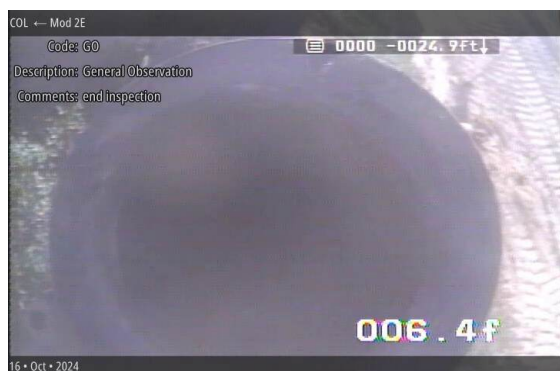
General Observation at 000.0 ft | end inspection
