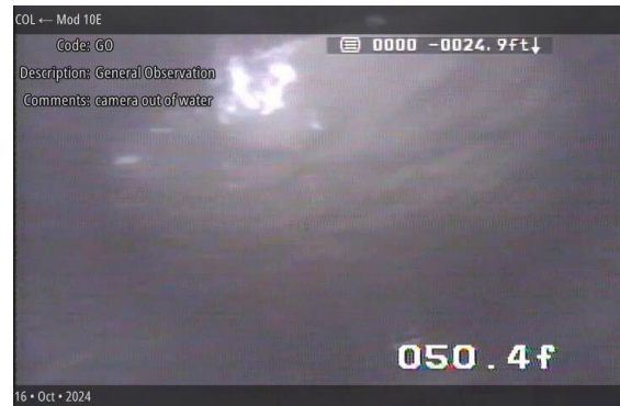
General Observation at 050.4 ft | camera out of water
