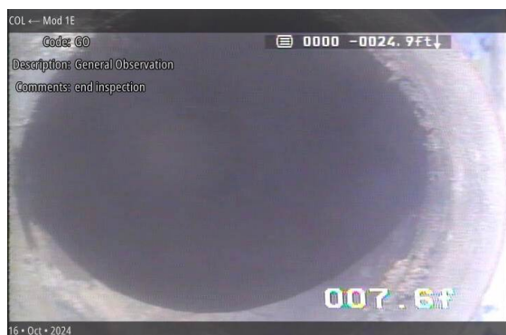
General Observation at 000.0 ft | end inspection
