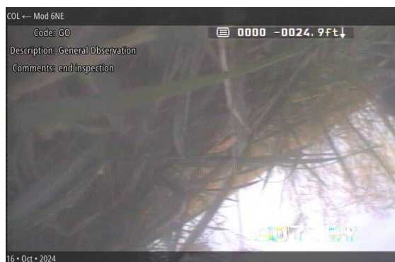
General Observation at 000.0 ft | end inspection
