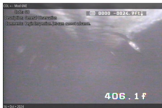
General Observation at 406.1 ft | Begin Inspection. Jet-cam cannot advance.
