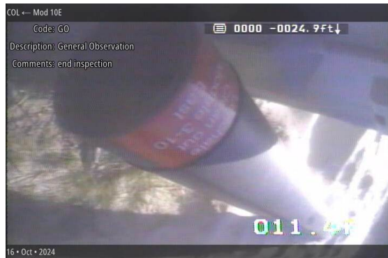
General Observation at 000.0 ft | end inspection
