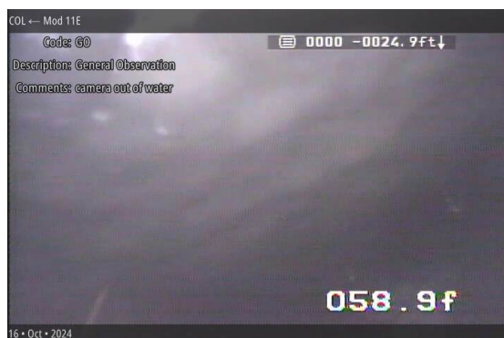
General Observation at 058.9 ft | camera out of water
