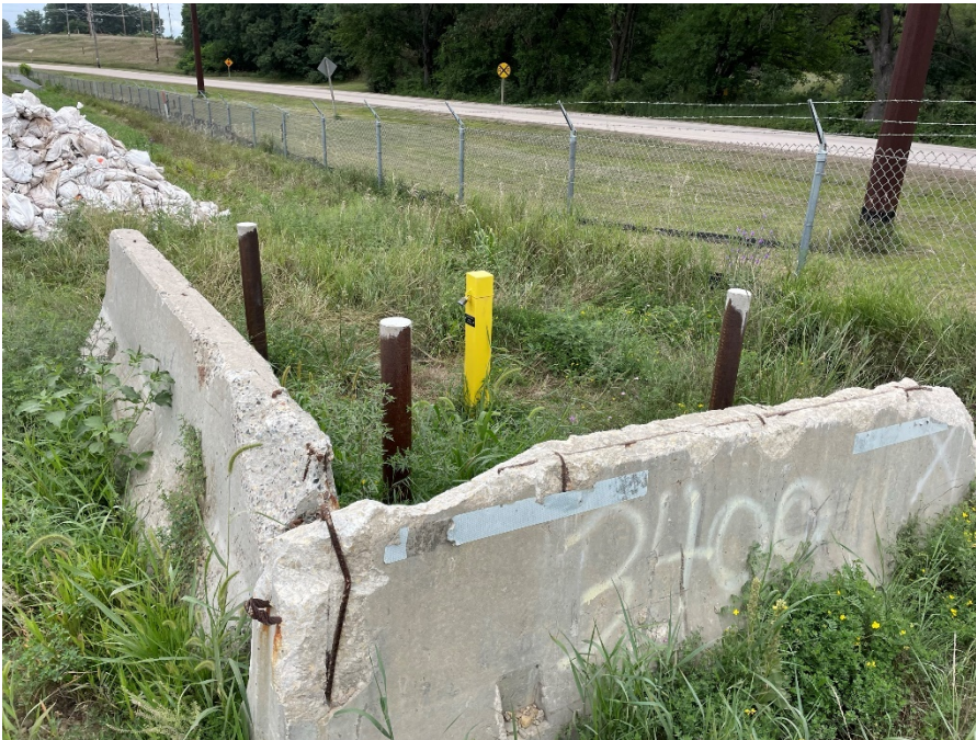
Photo 2: MW-318, looking northwest.
