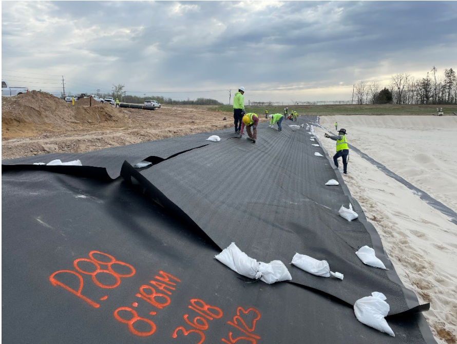
Photo 27: Placing geomembrane panels on the north berm of Module 11. (Looking east) (5/5/2023)
