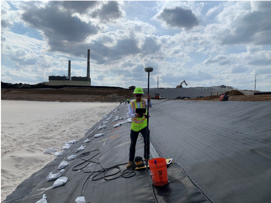
Photo 30: Surveying the geomembrane panels and repairs. (Looking west) (5/5/2023)
