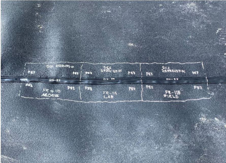
Photo 25: Marking and collecting destruct geomembrane samples. (Looking down) (5/4/2023)
