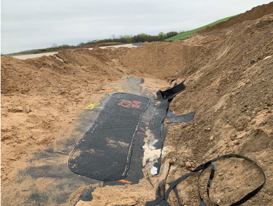
Photo 31: Repaired damaged section on the existing geomembrane of Module 4. (Looking south) (5/6/2023).
