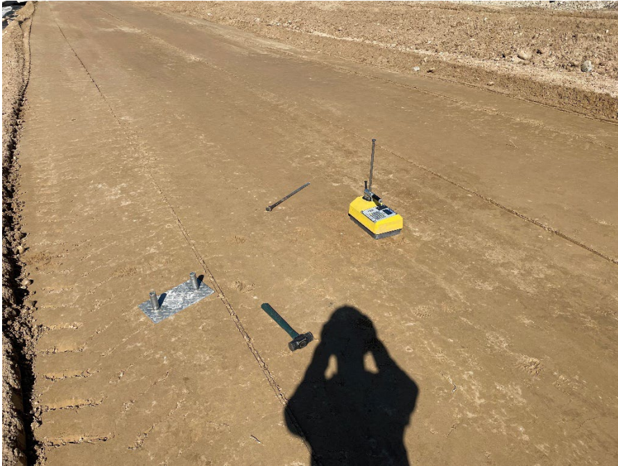
Photo 3: SCS NDG testing the general fill lifts for compaction. (Looking down) (4/13/2023)
