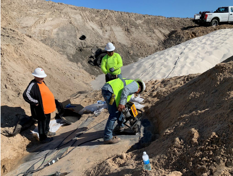
Photo 41: Geomembrane repairs between Modules 4 and 11. (Looking north) (5/20/2023)
