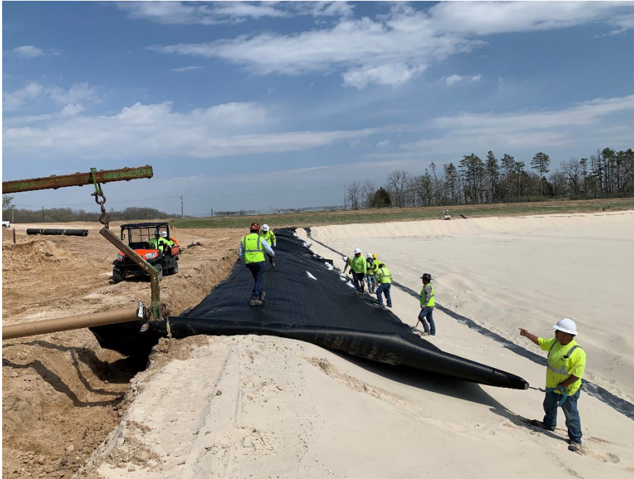
Photo 23: Installing geomembrane panels on the north berm of Module 11. (Looking east) (5/4/2023)
