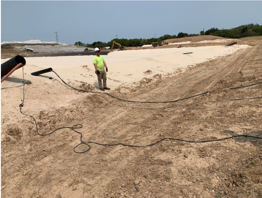
Photo 39: Re-televising the leachate collection pipes in Modules 10 and 11. (Looking northwest) (5/18/2023)
