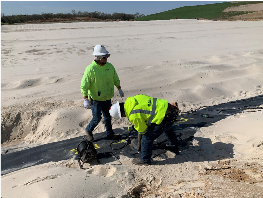
Photo 20: Performing geomembrane trial welds before seaming temporary geomembrane flap. (Looking southwest) (5/4/2023)
