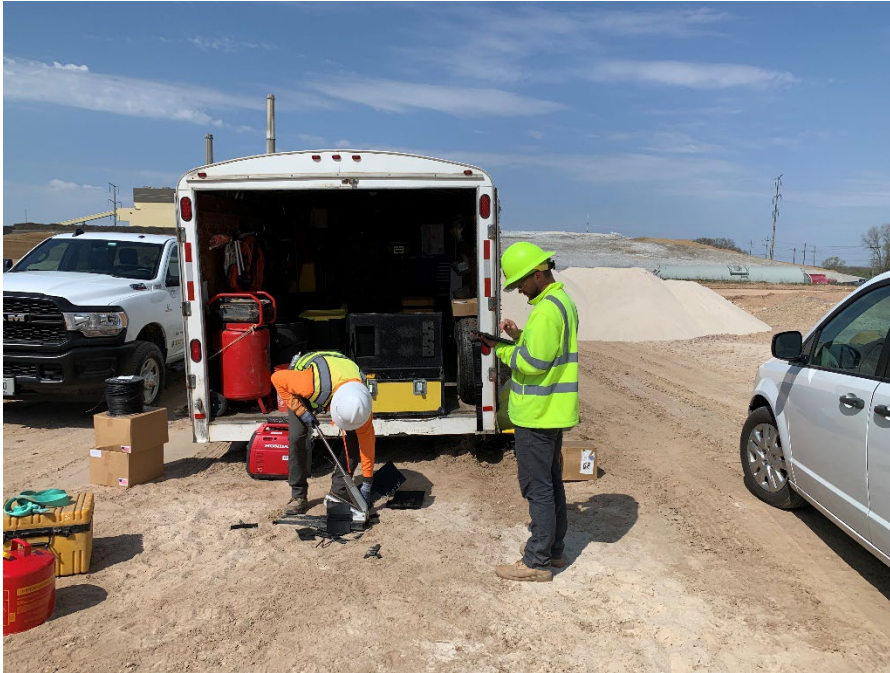
Photo 21: Field testing of the geomembrane trial welds. (Looking west) (5/4/2023)
