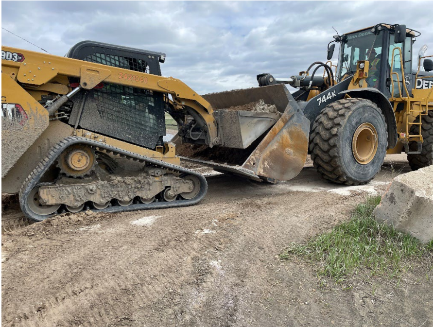
Photo 13: Mixing bentonite and sand mix for leachate header trench plugs. (5/2/2023)
