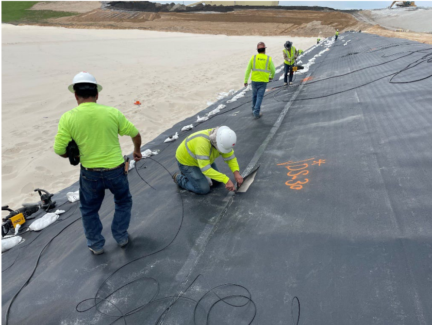
Photo 28: Collecting geomembrane destruct samples. (Looking west) (5/5/2023)
