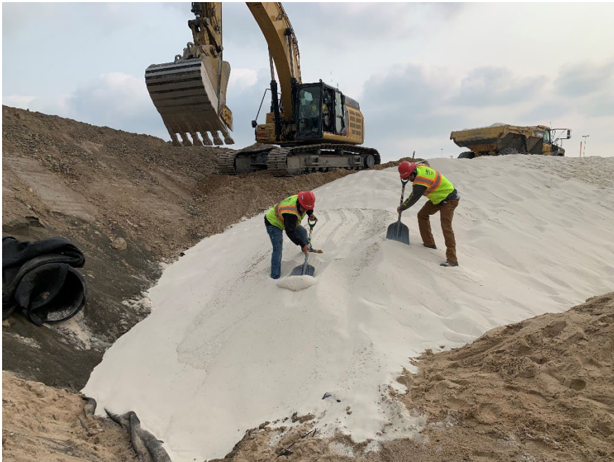
Photo 40: Finalizing the drainage material placement on the north berm. (Looking northeast) (5/19/2023)
