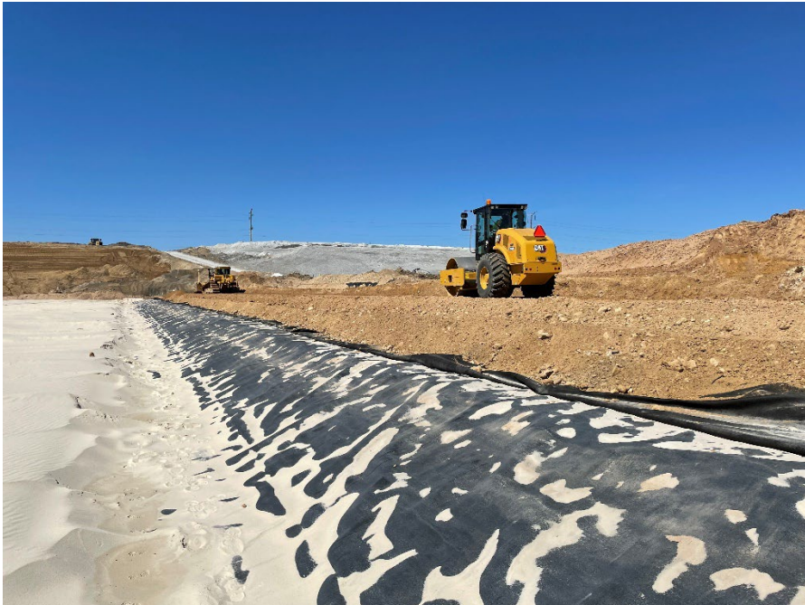
Photo 2: Compacting the general fill material for Module 11 northern berm. (Looking northwest) (4/13/2023)
