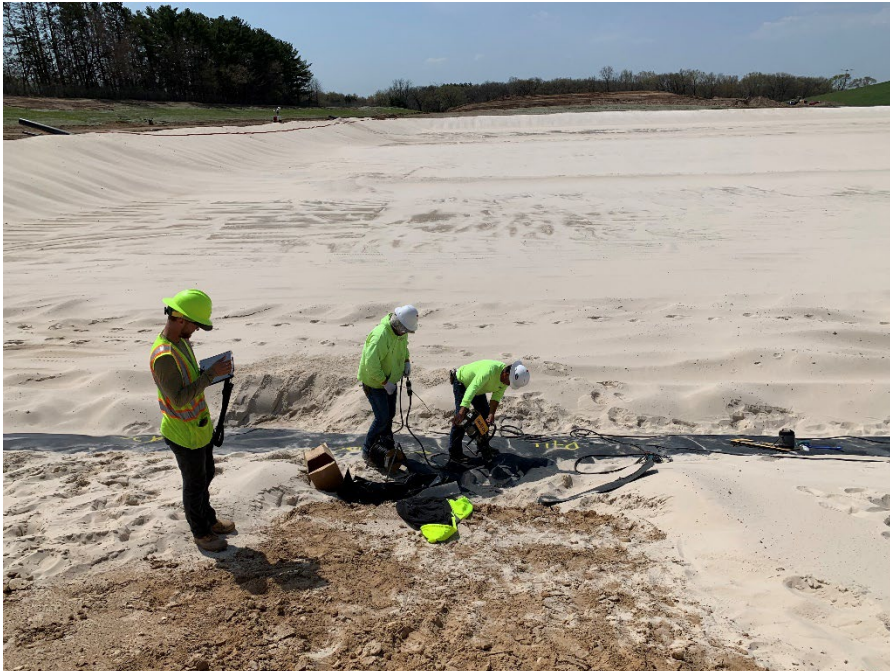
Photo 22: Repairing existing damage of the existing geomembrane. (Looking south) (5/4/2023)
