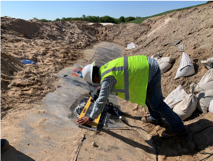
Photo 42: Vacuum box testing of the geomembrane repairs. (Looking south) (5/20/2023)
