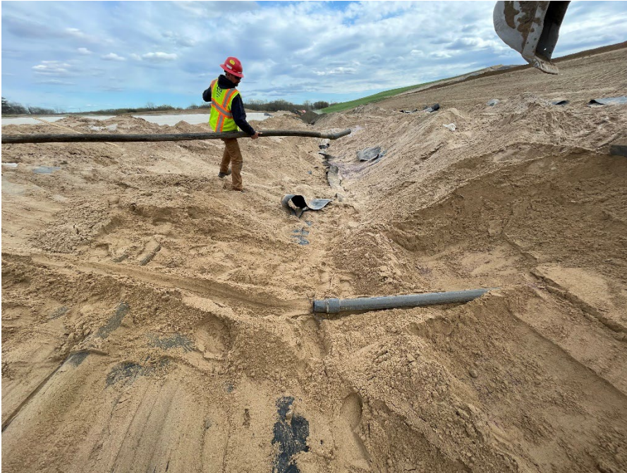
Photo 17: Removing the leachate headwell risers in both Modules 3 and 4. (Looking south) (5/3/2023)
