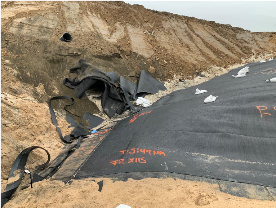
Photo 32: Northwest corner of Module 11 berm welded to existing flap of Module 5. (Looking northeast) (5/6/2023)
