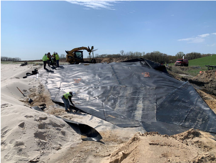
Photo 24: Placing geomembrane panels in the southwest corner of Module 10. (Looking south) (5/4/2023)
