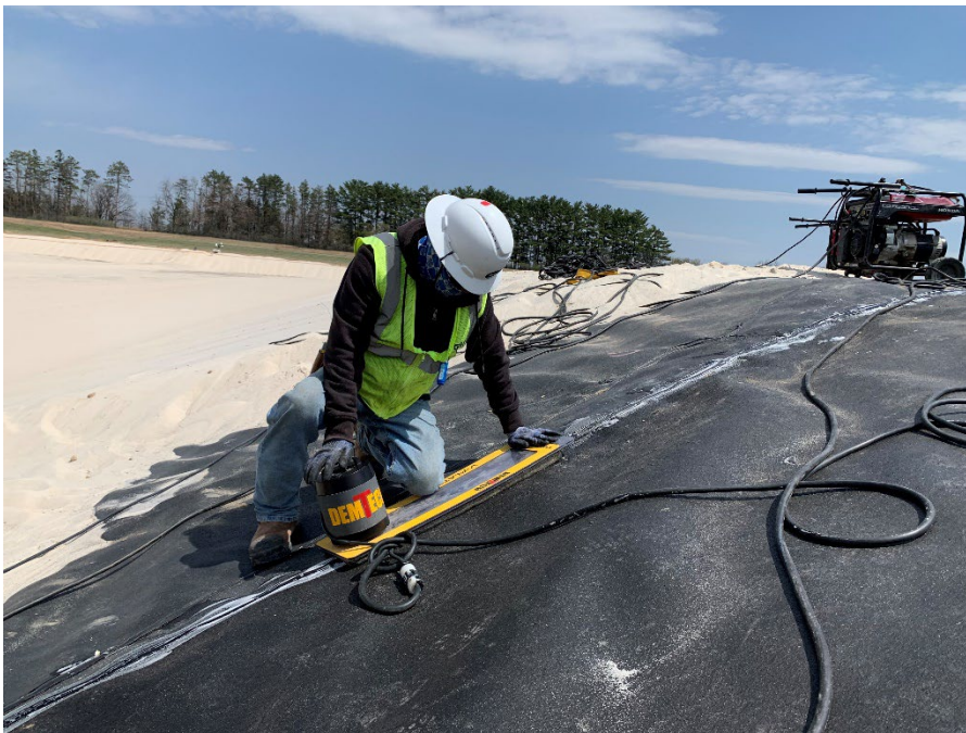
Photo 26: Vacuum box testing of extrusion seams. (Looking east) (5/4/2023)
