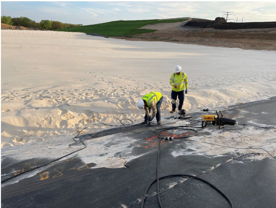
Photo 34: Collecting an additional destruct and performing repairs. (Looking southwest) (5/11/2023)
