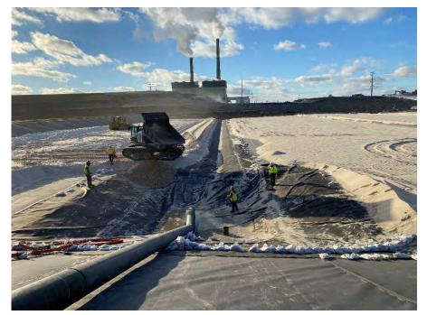
**Photo 91:** Placing coarse aggregate pipe bedding in Module 10 sump. (Looking west, 11/30/22).
