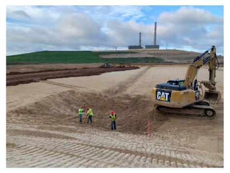
**Photo 32:** Excavating and grading the subgrade for the leachate collection sump in Module 10. (Looking west, 09/21/22).
