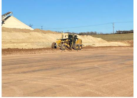
**Photo 67:** Final clay grading at Module 11 north berm. (Looking northeast, 11/01/22).
