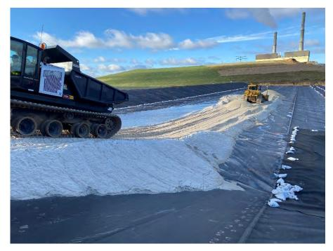
**Photo 82:** Tracked trucks placing and low-pressure dozer grading drainage material into Module 10 using haul road. (Looking west, 11/11/22).
