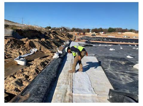
**Photo 70:** Tie-in the GCL in Module 10. (Looking north, 11/01/22).
