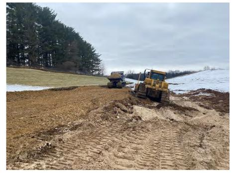
**Photo 107:** Placing and grading breaker run on perimeter access road. (Looking south, 12/12/22).
