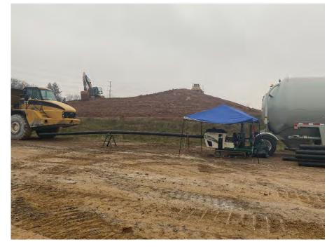
**Photo 88:** Fusing 6" HDPE leachate collection pipes. (Looking east, 11/29/22).
