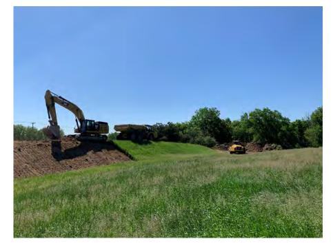
**Photo 4:** Stripping topsoil on the east berm, south of the leachate/surface water pond. (Looking southeast, 6/2/22).
