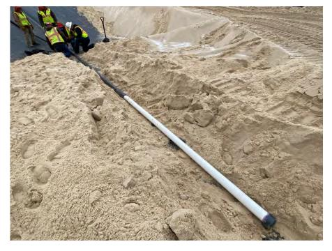
**Photo 97:** Leachate headwell pipe placed south of Module 11. (Looking down, 12/05/22).
