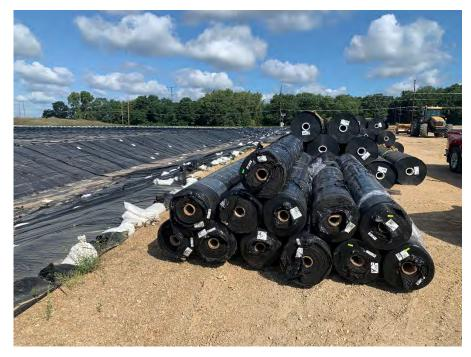
**Photo 28:** Geotextile seperator rolls delivered to the site. (Looking north, 09/06/22).
