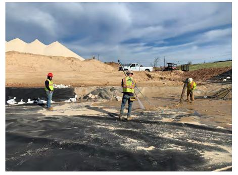
**Photo 79:** Badger Daylighting using water and a vacuum hose to clean up sediment on geomembrane liner from rain event. (Looking northeast, 11/08/22).
