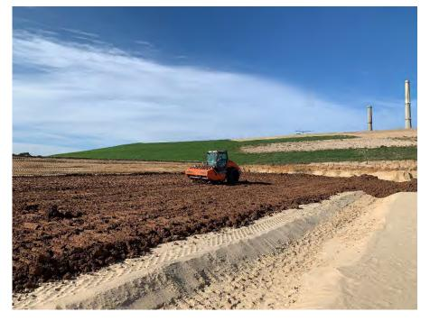
**Photo 35:** Compacting the clay material in Module 10 using the sheepsfoot compactor. (Looking southwest, 09/21/22).
