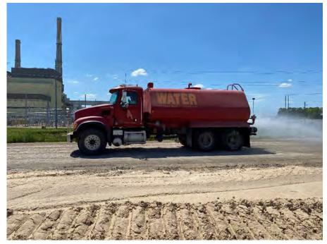
**Photo 16:** Using water truck for dust control onsite. (Looking northwest, 6/24/22).
