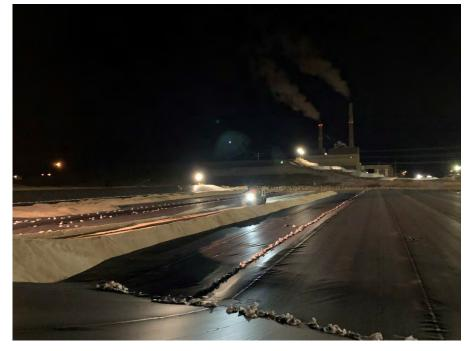
**Photo 83:** Placing drainage layer material in Module 10. (Looking west, 11/13/22).
