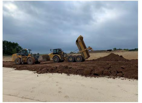
**Photo 31:** Placing clay in Module 10. (Looking southeast, 09/20/22).
