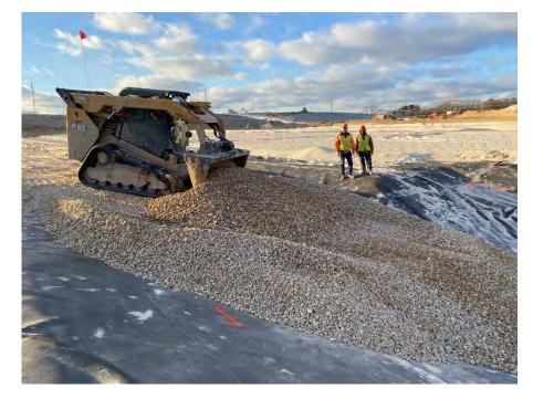
**Photo 92:** Grading pipe bedding material into the Module 10 sump area. (Looking northwest, 11/30/22).
