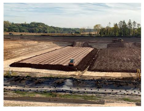
**Photo 48:** Compacting and sealing clay at the north half of Module 11. (Looking east, 10/05/22).
