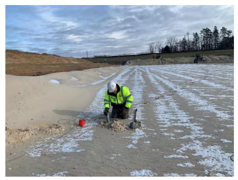
Photo 102: CQM conducting electrical leak location testing for Modules 10 and 11 geomembrane. (Looking east, 12/08/22).
