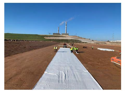
**Photo 58:** First day of geosynthetics. GSI placing GCL material south of Module 10 (Looking west, 10/29/22).
