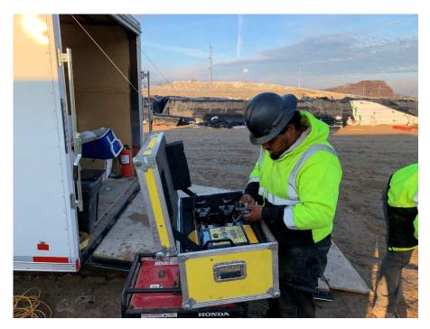
**Photo 5:** Testing the trial weld for the geommebrane. (Looking west, 10/28/22).
