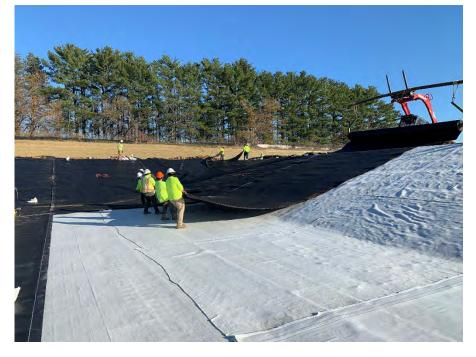
**Photo 60:** Placing geomembrane panels south of Module 10. (Looking southeast, 10/29/22).
