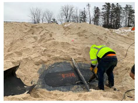
**Photo 111:** GSI performing extrusion geomembrane seaming for the repairs. (Looking east, 12/13/22).
