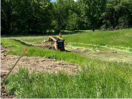
**Photo 10:** Adding stone check at the southwest corner of the proposed stockpile area. (Looking southwest, 6/9/22).
