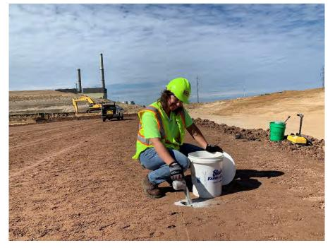
**Photo 45:** Filling holes created in the clay (due to the moisture/density tests and collecting Shelby tube) with granular bentonite. (Looking west, 10/03/22).
