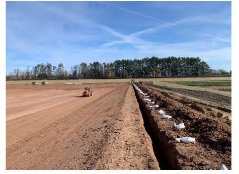
**Photo 57:** Smooth drum rolling the clay surface of Module 10, and GSI staging sandbags for geosynthetics. (Looking east, 10/28/22).
