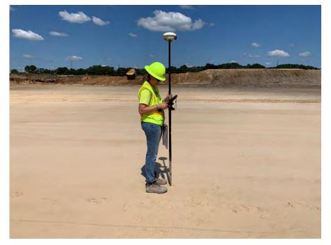
**Photo 25:** SCS surveying subbase documentation points in Module 10. (Looking north, 8/23/22).
