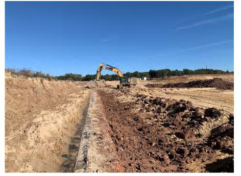
**Photo 49:** Exposing and creating clay step into existing clay from Modules 3 and 4. (Looking north, 10/08/22).
