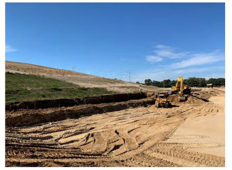
**Photo 43:** Excavating overburden material to expose the tie-in to Modules 3 and 4 on west end of Module 10. (Looking northwest, 09/30/22).
