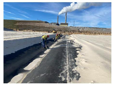
**Photo 93:** Cleaning sand off of the leachate collection trenches before placing coarse aggregate pipe bedding. (Looking west, 12/01/22).
