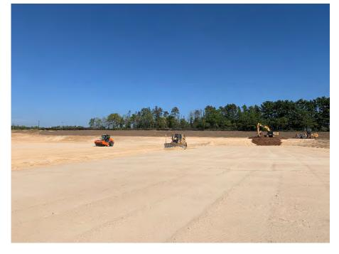
**Photo 30:** Final grading of subbase in Module 10. (Looking east, 09/19/22).
