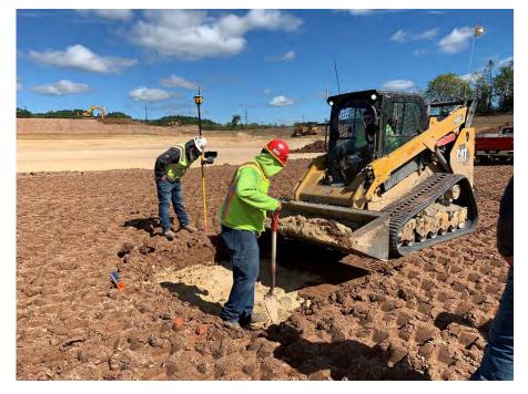
**Photo 37:** Removing clay mixed with sand from the first lift. (Looking northeast, 09/22/22).
