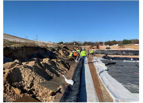
**Photo 69:** Exposing the existing Module 3 GCL material for tie-in with Module 10 material. (Looking north, 11/01/22).
