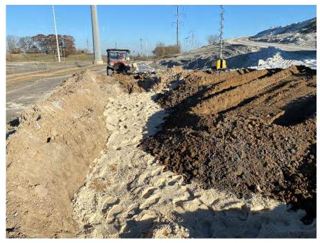
**Photo 12:** Repair area covered with 1 foot of COVIA sand drainage material and backfilled with clean general fill. (Looking north, 11/02/22).
