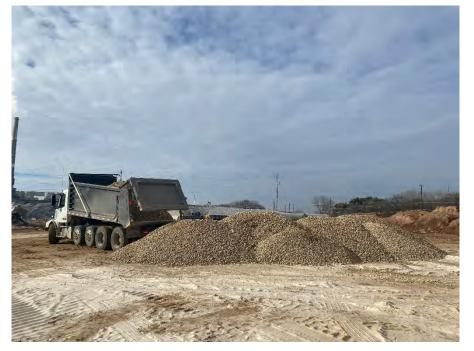
**Photo 85:** Coarse aggregate pipe bedding delivered to the site. (Looking west, 11/22/22).
