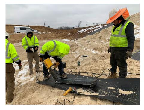
**Photo 108:** Performing extrusion trial welds for the geomembrane before completing the repairs that were located by the leak location test. (Looking northeast, 12/13/22).
