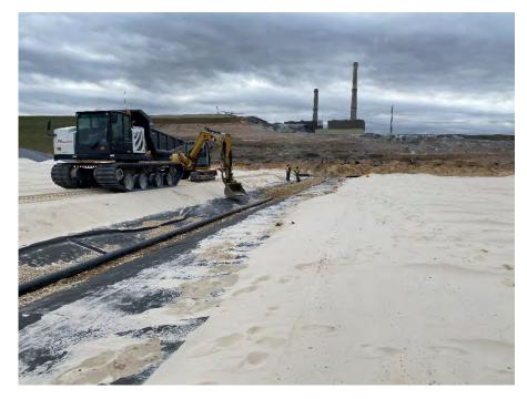
**Photo 96:** Placing coarse aggregate pipe bedding using haul roads adjacent to the leachate collection trench in Module 10. (Looking west, 12/02/22).
