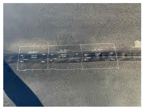
**Photo 76:** Marked destructive test location for fusion welds. (Looking down, 11/07/22).
