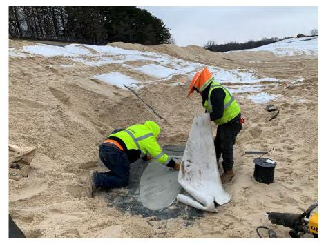
**Photo 110:** GSI fixing GCL locations at the geomembrane repair areas. (Looking south, 12/13/22).
