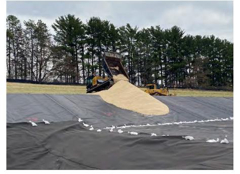
**Photo 81:** Tracked haul trucks placing drainage material to form 2' thick ramp into Module 10. (Looking southeast, 11/10/22).
