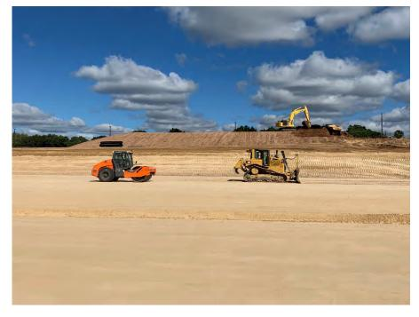
**Photo 38:** Grading and compacting subbase in Module 11. Background: excavating clay from the onsite stockpile. (Looking north, 09/22/22).
