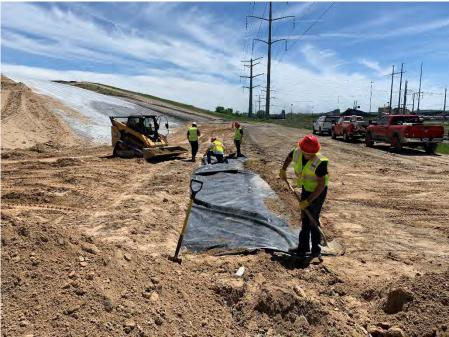
**Photo 2:** Placing a (~18'x~25') section of rain cover material to prevent water from migrating under the geomembrane liner. (Looking south, 6/2/22).
