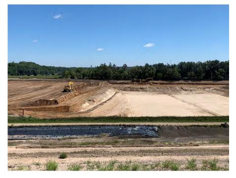
**Photo 26:** View of Module 10 subbase and excavation process of the overburden material in Module 11. (Looking east, 08/30/22).
