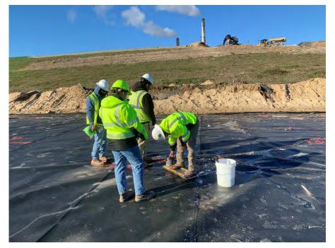
**Photo 77:** GSI performing vacuum box tests for extrusion seams. (Looking west, 11/07/22).
