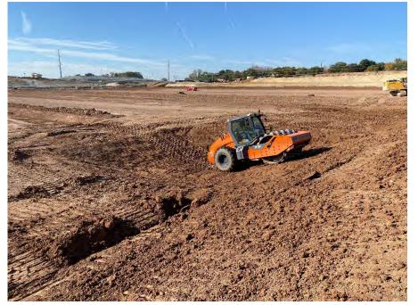
**Photo 53:** Compacting clay lift in Module 10 sump. (Looking northwest, 10/20/22).
