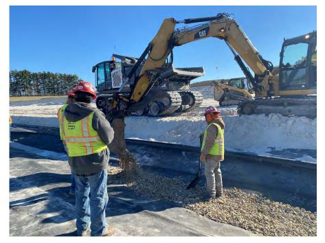
**Photo 94:** Placing coarse aggregate pipe bedding in the leachate collection trenches. (Looking southeast, 12/01/22).
