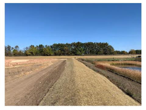
**Photo 50:** Highway Landscapers placing erosion mat on berm north of the leachate/surface water pond and on east perimeter slopes. (Looking east, 10/10/22).
