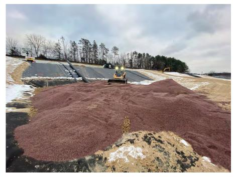
**Photo 101:** Grading filter material in Module 11 sump. (Looking southeast, 12/07/22).
