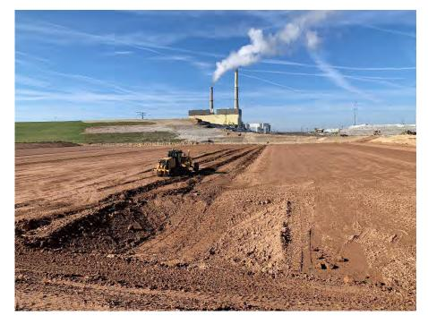
**Photo 54:** Grading base grade in Module 11. (Looking west, 10/27/22).
