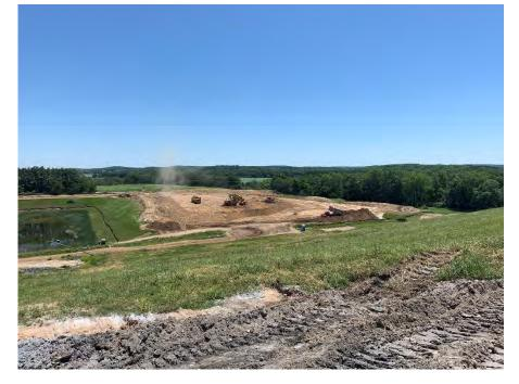
**Photo 14:** Stockpiling excavated overburden material and topsoil. (Looking southeast, 6/23/22).
