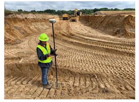
**Photo 21:** Excavating overburden material from the west side of Module 10. Checking subbase grades. (Looking north, 8/15/22).
