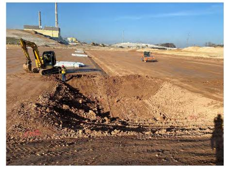
**Photo 65:** Grading base grade for Module 11 sump. (Looking west, 10/31/22).
