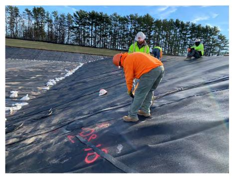
**Photo 78:** Repairing the location of destructive geomembrane sample. (Looking east, 11/08/22).
