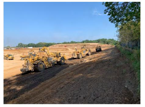
**Photo 29:** Placing topsoil at the east slope, east of Modules 10 and 11. (Looking north, 09/16/22).
