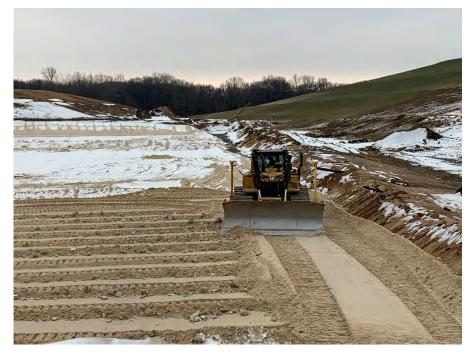
**Photo 114:** Connecting drainage layers between Modules 11 and 4. (Looking south, 12/13/22).
