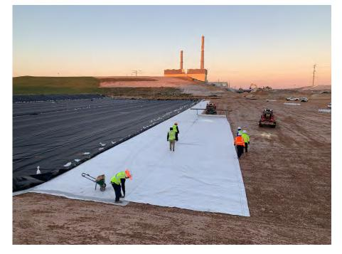
**Photo 72:** Placing GCL panels south of Module 11 (Looking west, 11/02/22).
