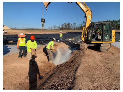
**Photo 71:** Placing additional bentonite to smooth Module 10 leachate collection trench. (Looking east, 11/01/22).
