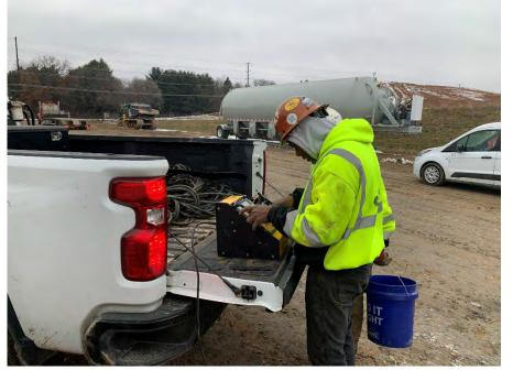
**Photo 109:** Testing geomembrane trial welds using the field tensiometer. (Looking northeast, 12/13/22).
