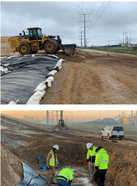
Photo 3: Adding general fill material to the west end of Mod 4-5 haul road to protect the liner. (Looking south, 6/11/22).
