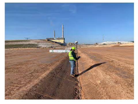
**Photo 66:** SCS surveying documentation points in Module 11 leachate collection trench. (Looking west, 10/31/22).
