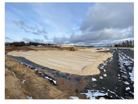
**Photo 84:** Low-groundpressure bulldozer (CAT-D6T LGP) grading drainage layer into 1' thickness in Module 11. (Looking northeast, 11/16/22).
