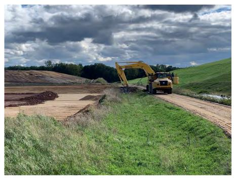
**Photo 40:** Stripping topsoil from the swale west of Modules 10 and 11. (Looking south, 09/26/22).
