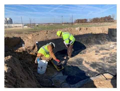
**Photo 11:** GSI vacuum box testing extrusion weld. (Looking northwest, 10/28/22).
