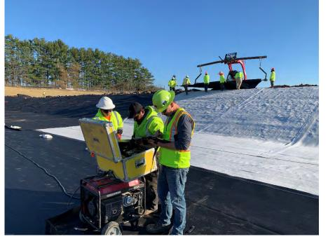
**Photo 61:** Testing geomemebrane trial welds using the field tensiometer. (Looking southeast, 10/29/22).
