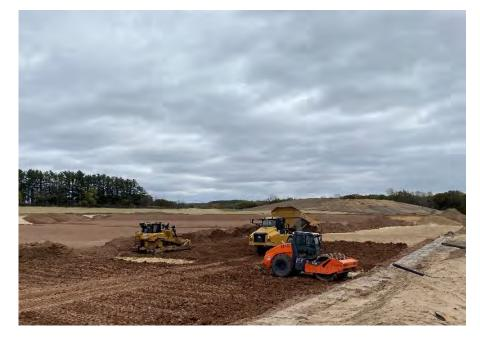
**Photo 52:** Placing, grading, and compacting lift of clay step at the west end of Modules 10 and 11. (Looking southeast, 10/17/22).
