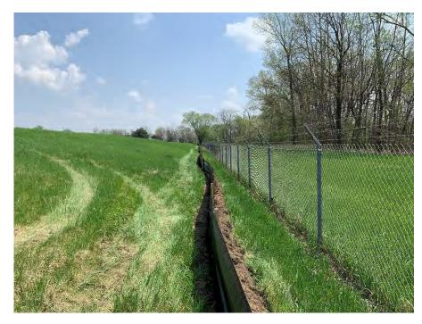
**Photo 2:** Highway Landscapers installed silt fence south of the proposed location of the overburden stockpile along the chain-link fence (Looking east, 5/12/22).
