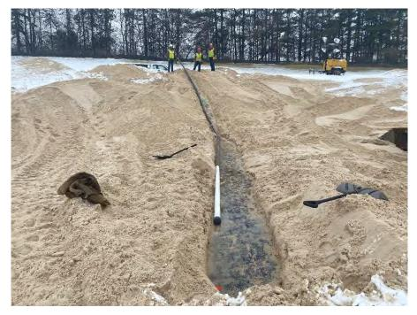
**Photo 105:** Leachate head well placed south of Module 10. (Looking east, 12/10/22).
