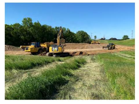
**Photo 6:** Stripping and stockpiling topsoil at the proposed stockpile area. (Looking south, 6/3/22).
