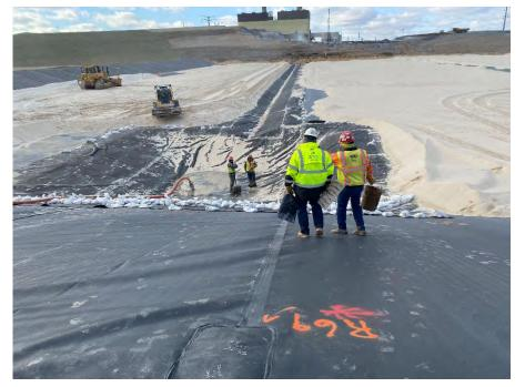
**Photo 89:** Ames laborers using plastic shovels to remove blown-in sand from geotextile cushion surface in sump area. (Looking west, 11/30/22).
