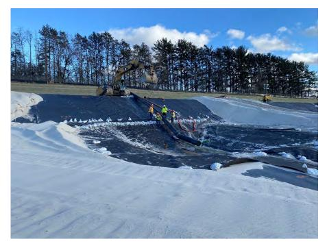
**Photo 90:** Placing 18" HDPE leachate collection piping sump pipe in Module 10. (Looking southeast, 11/30/22).
