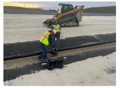
**Photo 95:** Fusing 6" HDPE leachate collection pipes. (Looking southwest, 12/01/22).
