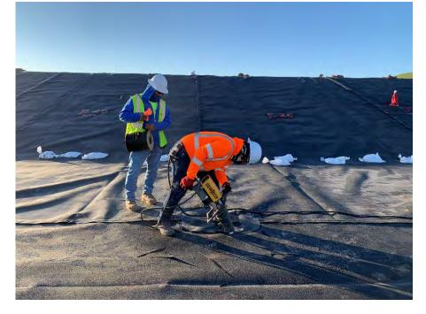
**Photo 68:** Performing extrusion welding for the geomembrane repairs. (Looking south, 11/01/22).
