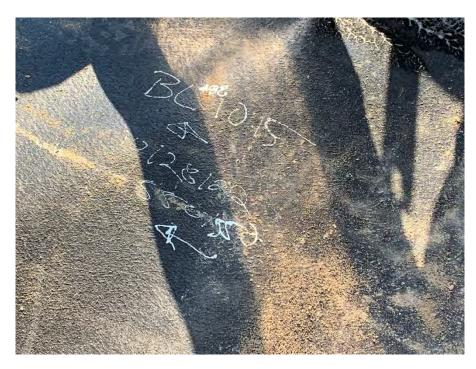
**Photo 9:** GSI recording the welder and machine information after completing the extrusion weld. (Looking down, 10/28/22).
