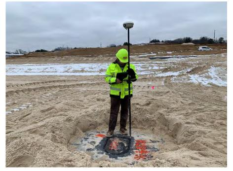
**Photo 113:** SCS surveying the locations of the geomembrane repairs. (Looking north, 12/13/22).
