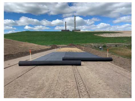
**Photo 39:** Placing geotextile separator and breaker run for the access road north of the overburden stockpile (Looking west, 09/22/22).
