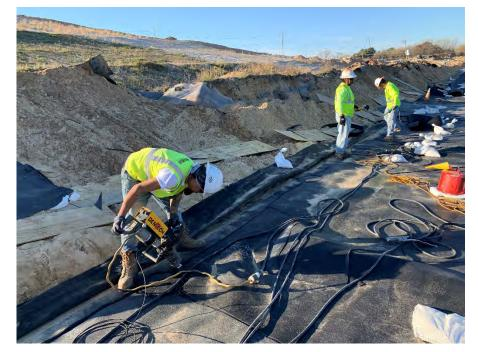
**Photo 75:** Extrusion welding for the geomembrane tie-in between Module 10 and Module 3. (Looking northwest, 11/02/22).
