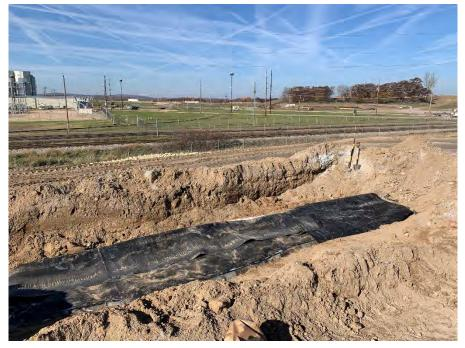
**Photo 10:** View of the repair after completion. West portion of the repair was placed in the anchor trench. (Looking northwest, 10/28/22).
