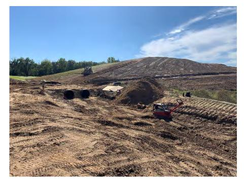
**Photo 44:** Installing 30-inch HDPE culverts southeast of Module 10. (Looking southwest, 09/30/22).
