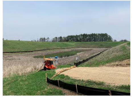
**Photo 1:** Highway Landscapers installed a sediment log across the leachate/surface water pond access road, and silt fence around the leachate/surface water pond (Looking northeast, 5/11/22).
