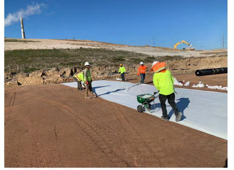
**Photo 59:** Placing bentonite for the overlap edges of the GCL material. (Looking northwest, 10/29/22).
