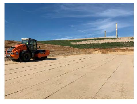
**Photo 22:** Smoothing subbase in the south area of Module 10. (Looking west, 8/18/22).
