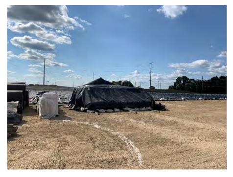
**Photo 24:** GCL rolls covered with rain cover (tarp) material. (Looking northwest, 8/23/22).
