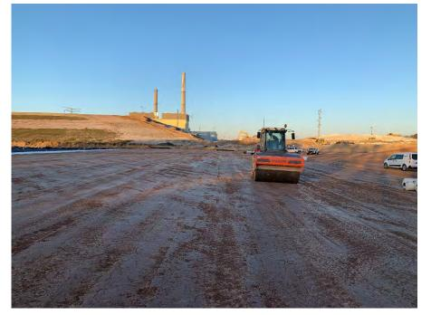
**Photo 73:** Smoothing the clay surface in Module 11 before geosynthetcs installation. (Looking west, 11/02/22).
