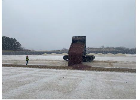
**Photo 99:** Placing filter material in Module 10 trench. (Looking south, 12/06/22).
