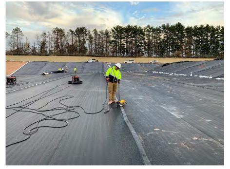
**Photo 63:** Fusion welding of the geomembrane seams. (Looking east, 10/30/22).
