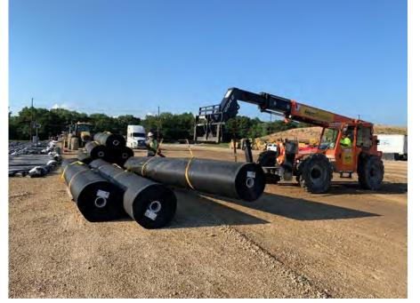
**Photo 19:** Geomembrane rolls delivered to the site. (Looking northeast, 8/10/22).
