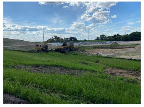
**Photo 11:** Stripping and hauling topsoil from Module 11 area. (Looking northwest, 6/9/22).
