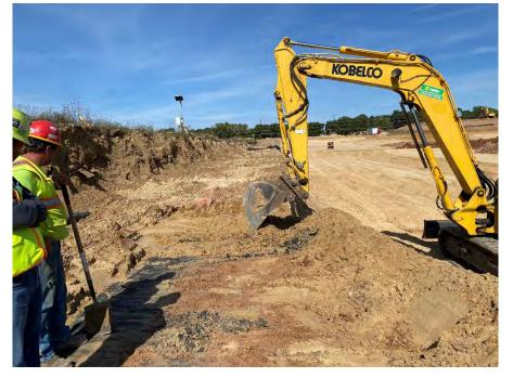
**Photo 47:** Exposing the existing clay liner of Modules 3 and 4 for tie-in. (Looking north, 10/04/22).
