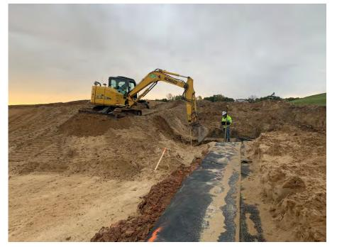
**Photo 51:** Excavating subbase and surveying documentation points in southwest corner of Module 10. (Looking south, 10/13/22).
