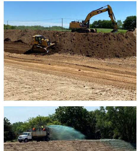
**Photo 17:** Placing topsoil in the swale east of the overburden material stockpile. (Looking southwest, 6/24/22).
