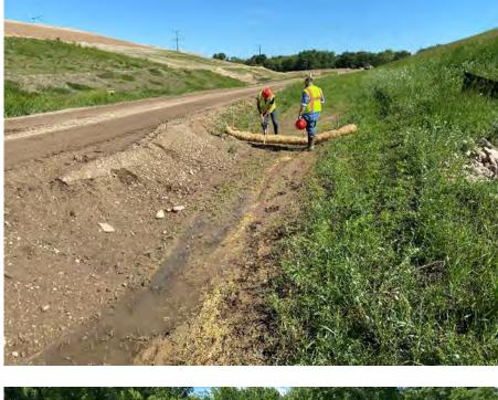
**Photo 9:** Adding sediment logs to the east swale, next to the leachate/surface water pond. (Looking north, 6/9/22).
