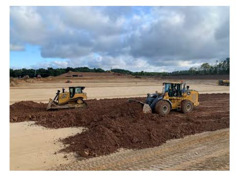
**Photo 34:** Spreading and grading the clay in Module 10. (Looking northeast, 09/21/22).
