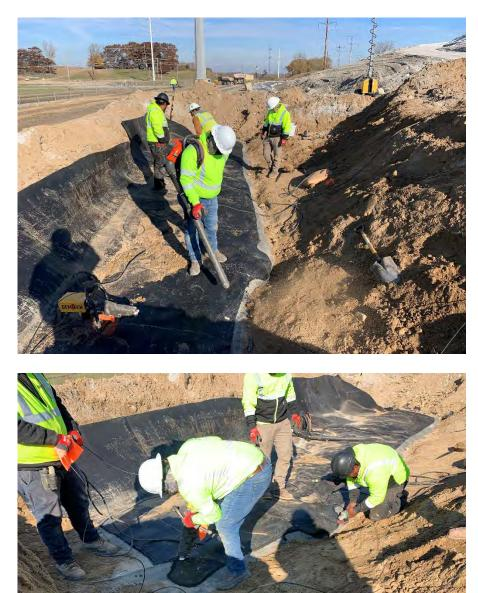
**Photo 7:** GSI removing sediment from welding area. (Looking north, 10/28/22).
