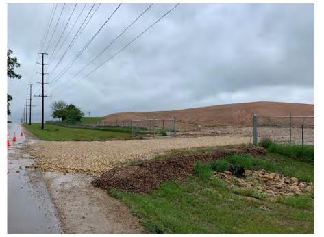
**Photo 7:** Completed tracking pad at the north entrance of the laydown area. (Looking southeast, 6/8/22)
