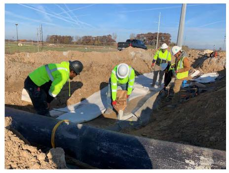
**Photo 6:** GSI placing granular bentoite before installation of new GCL. (Looking northwest, 10/28/22).
