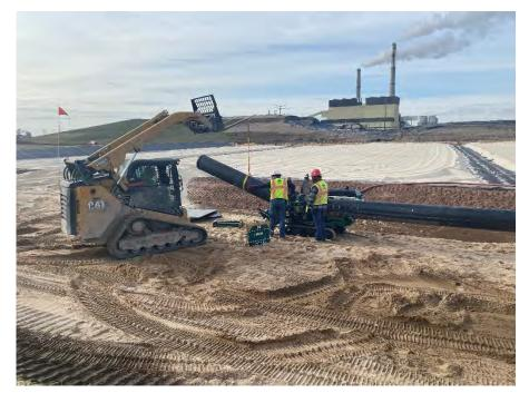
**Photo 86:** Fusing 18" leachate collection pipe. (Looking west, 11/28/22).
