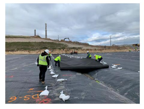
**Photo 80:** Placing geotextile cushion for the leachate collection trenches. (Looking west, 11/09/22).
