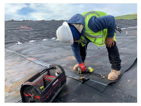
**Photo 64:** Air testing of the geomembrane fusion seams. (Looking southwest, 10/30/22).
