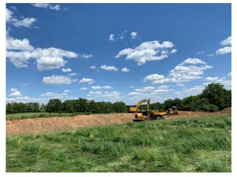
**Photo 5:** Excavating overburden material from the east berm, south of the leachate/surface water pond. (Looking southeast, 6/2/22).
