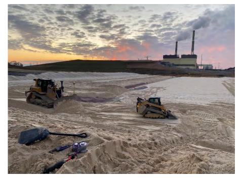
**Photo 103:** Grading drainage layer material in Modules 10 and 11 (Looking west, 12/08/22).
