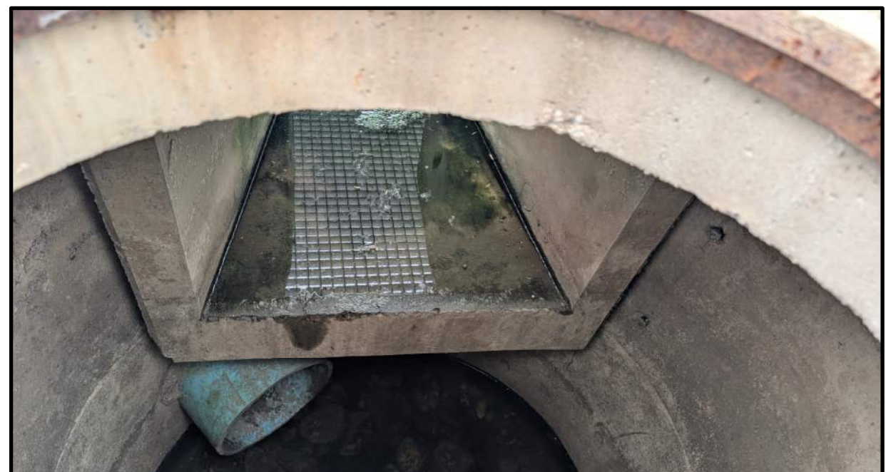
Inside Discharge Structure
