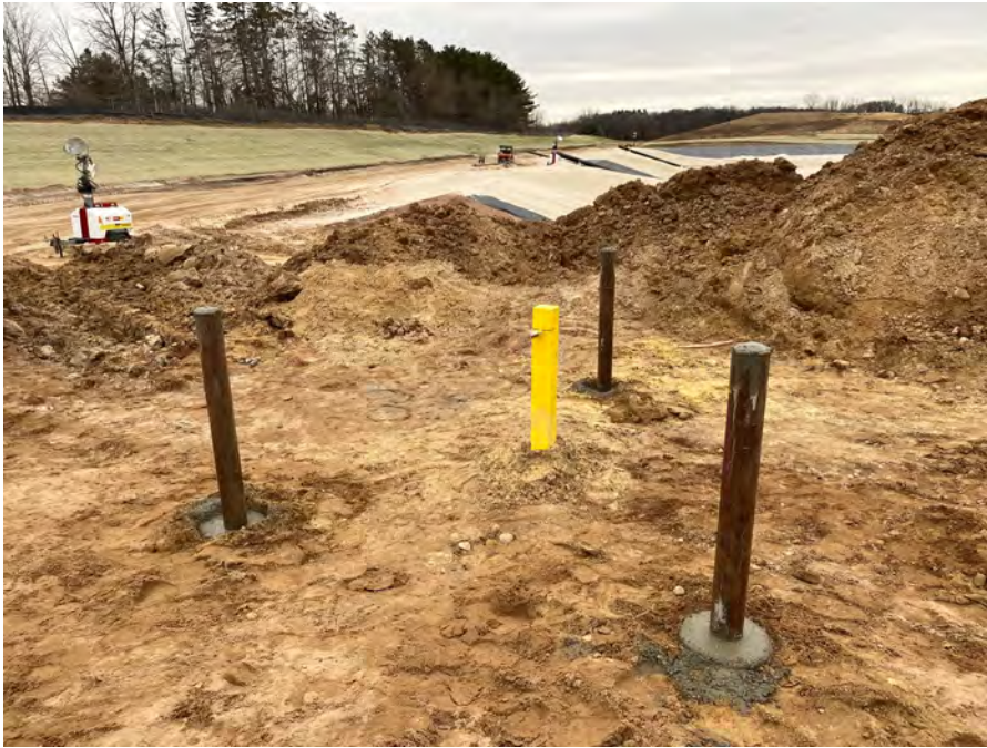
Photo 3: MW-315, looking southeast.
